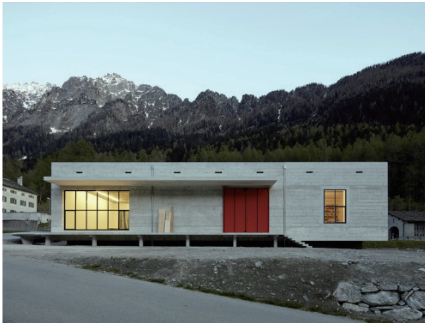
Magazzino & Atelier Miriam Cahn, Architect A. Ruinelli, Ansicht Nord, photograph@Ralph Feiner, 7208 Malans, CH, n.d.
